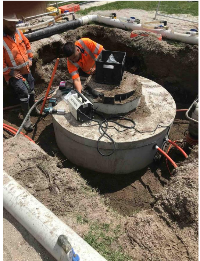
Completing the connections of the electrical conduits and discharge pressure line.
