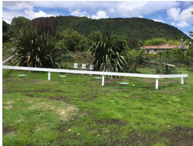
Rotoiti School System Install
