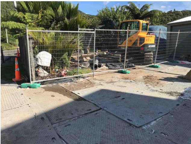
Onsite surface and security protections in place during the install
