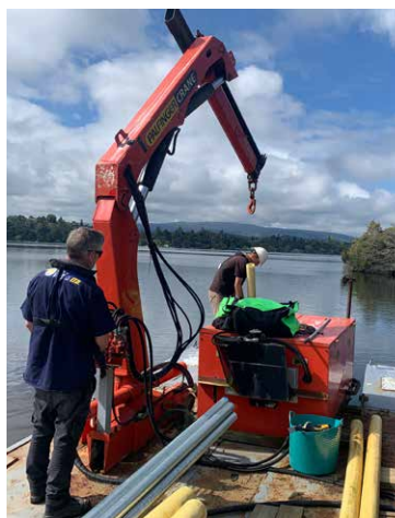
Straightening and resurfacing south cardinal.
